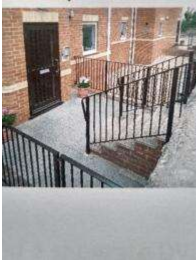
Front Entrance to Sandringham Court from High Street
